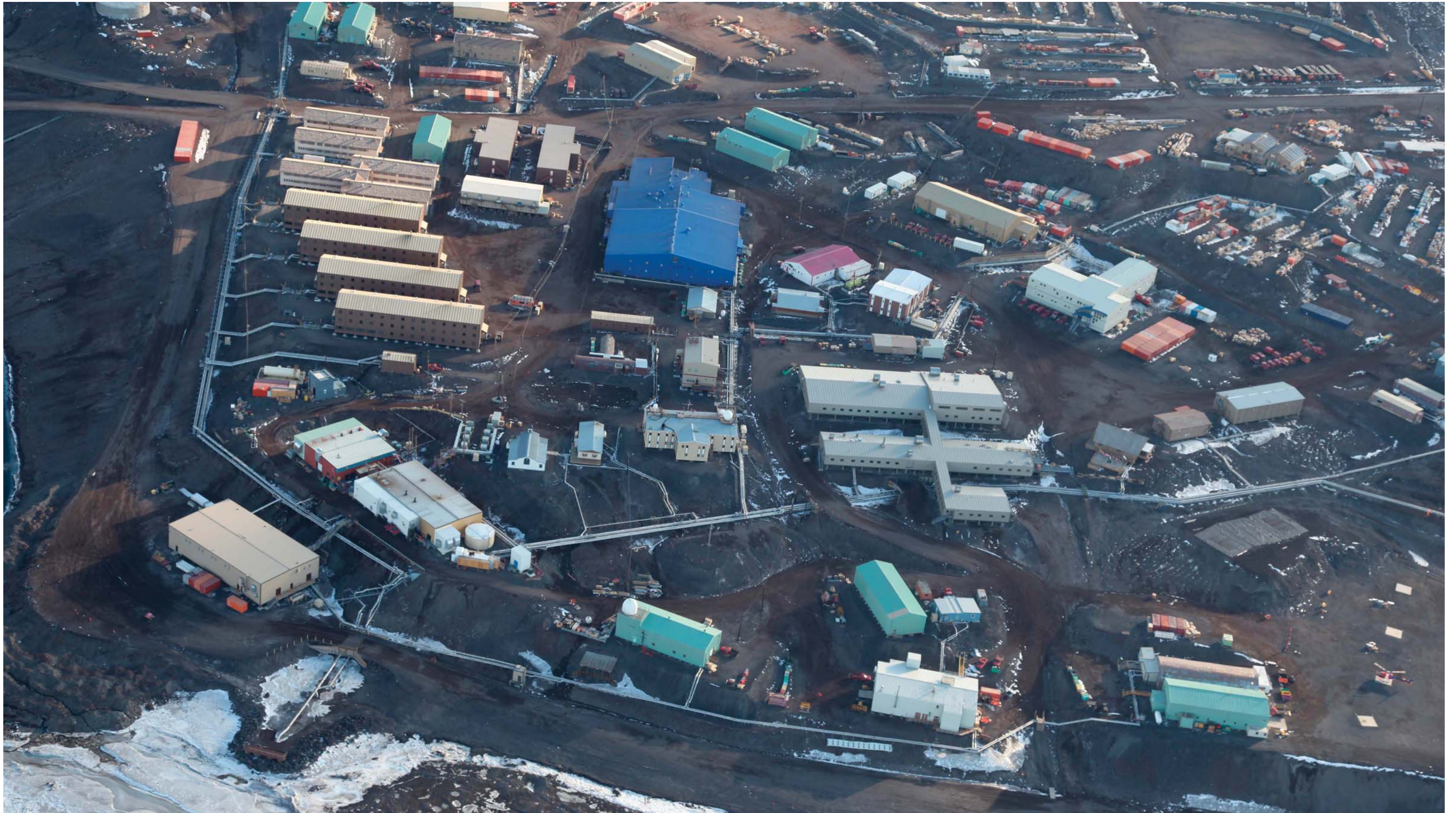
EXISTING MCMURDO STATION
